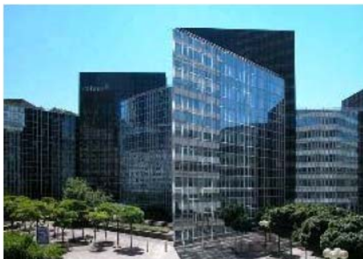
Tour Coface office building (Paris)
