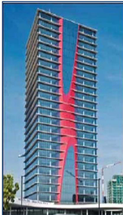
BCN office Tower (Barcelona)
